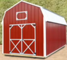
BRITE RED METAL SIDING WITH ALAMO WHITE TRIM AND METAL ROOF
